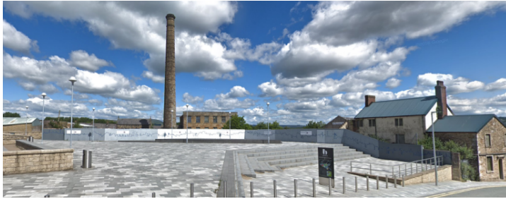
Existing Sandygate Square with Neptune Inn
