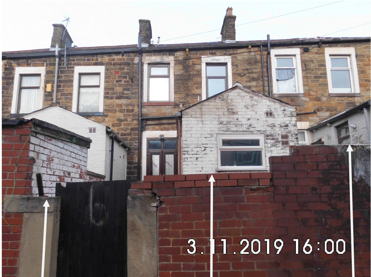
rear of no.8
